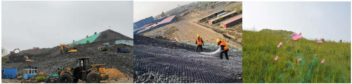
**Figure 2.** Vegetation coverage of Fengfeng mining area after spraying soil
