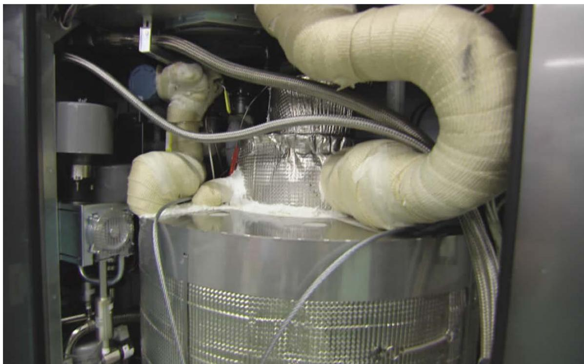
**Figure 7.** The inner structure of “Fridge” electricity station developed by Bloom Energy
