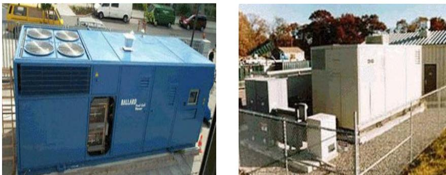
Figure 2. (left) Ballard Company 250 kW proton-exchange fuel cell stack and (right) the factory based on heat and power cogeneration system
