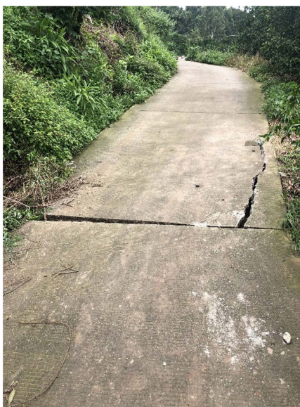
Figure 8. Transverse crack
