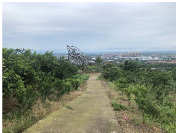
Figure 5. Broken tower 图 5. 铁塔折断
