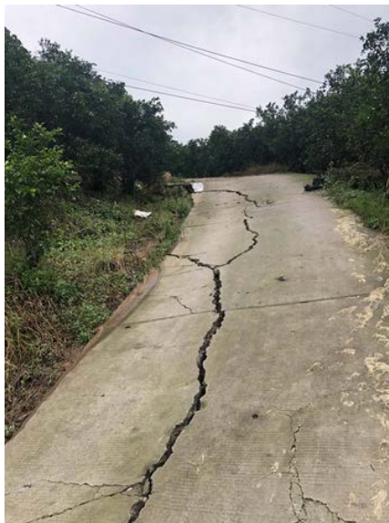
Figure 7. L-shaped crack
