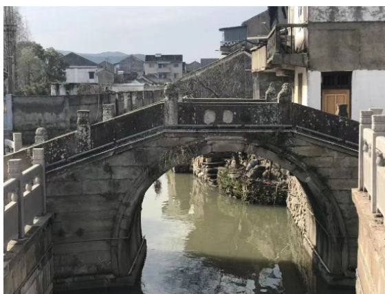
Figure 1. Doutang bridge 图1. 陡塘桥 ①
