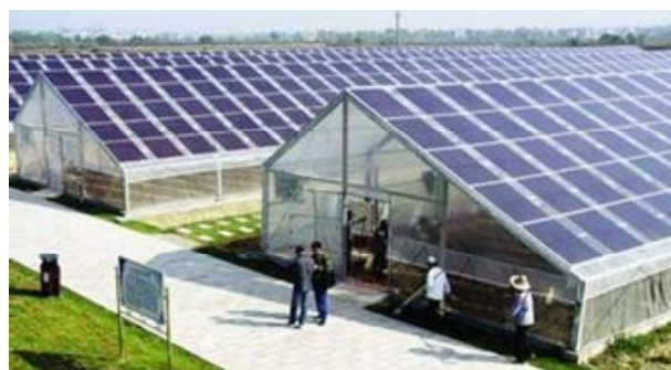
Figure 11. In order to install the fixed flat PV on the rooftop of the greenhouse, some designers used spacious gap between houses, which causes a waste of land 图 11. 为了克服光伏阵列的遮光问题，农业大棚只好以间隔的形式沿南北方向分开，使得土地使用率下降
