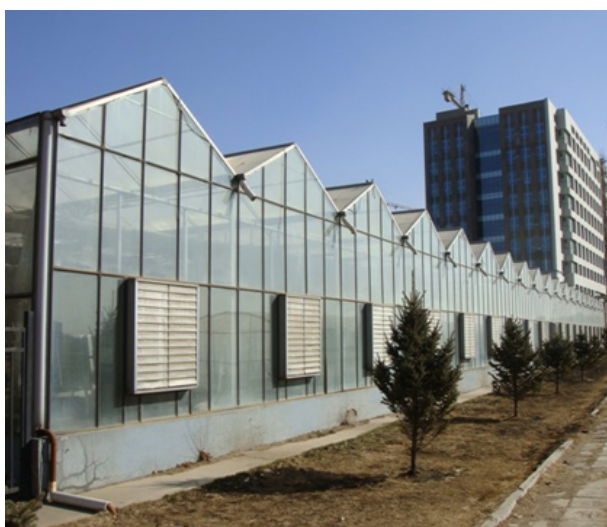
Figure 12. The greenhouse designed in the above case is inconvenient to install the fixed flat PV 图 12. 快速发展的能够与植物工厂相比美的密封式玻璃大棚不容易铺设固定式光伏电池
