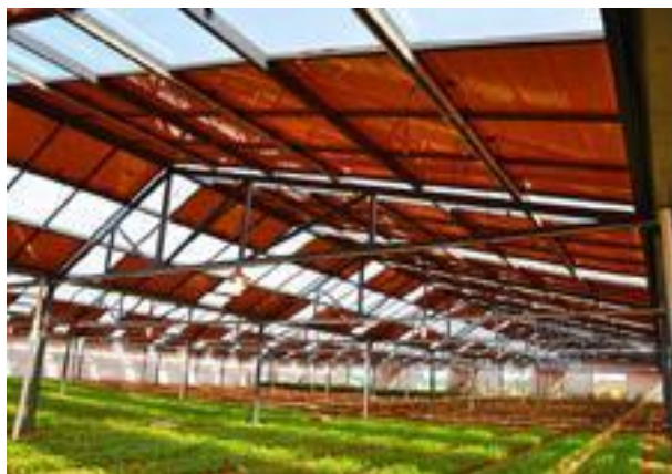
Figure 10. Any fixed flat PV installed on the rooftop of greenhouse will cause sacrifice of sunlight 图 10. 固定式平板光伏安装在农业大棚上会产生植物同光电争夺阳光的矛盾
