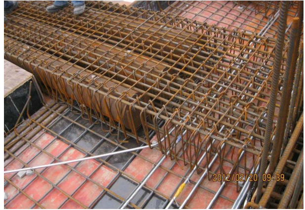
Figure 6. The connection diagram of hollow steel tube and wall cap 图 6. 空心钢管与墙帽连接图
