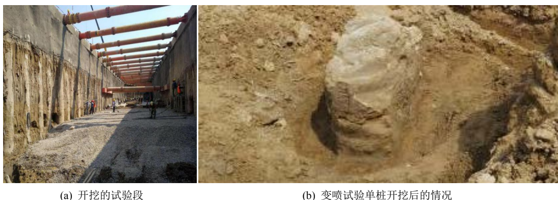
Figure 3. Rotary jet grouting test for the Zong-er municipal road underground pipe corridor project 图 3. 纵二路市政道路地下管廊工程变喷试验
