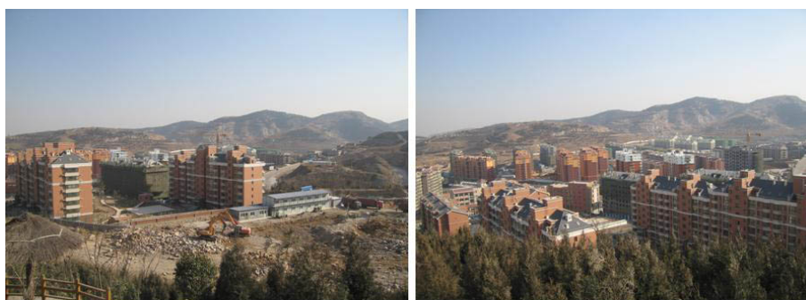
Figure 2. Urbanization status of construction and development in the karst mountainous region of Jinan City
