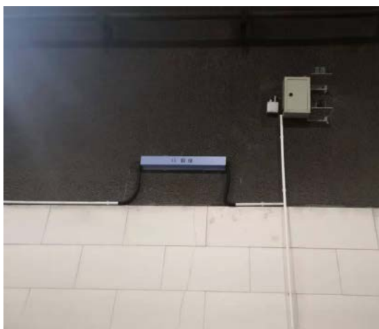
Figure 4. Detection site of bridge bottom 图 4. 桥底检测现场
