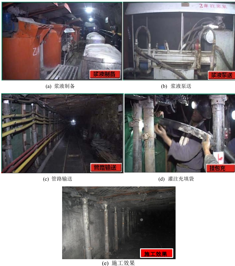
Figure 3. The process of reserving roadway with filling 图 3. 充填留巷过程
