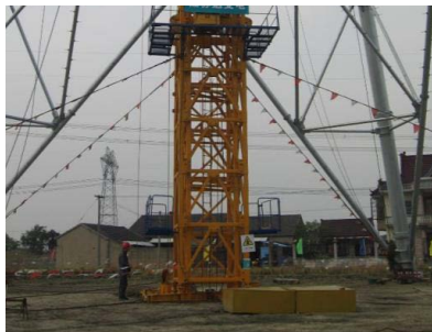
Figure 1. The under jacking mechanism 图 1. 下顶升机构
