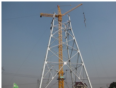
Figure 4. Erect tower of special-purpose tower crane 图 4. 专用塔机组塔
