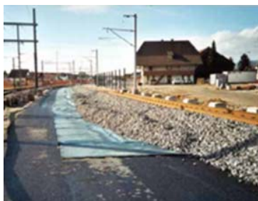
Figure 9. Under ballast mats 图 9. 道砟垫
