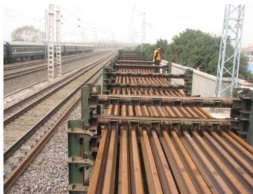
Figure 1. The photo of long rail car dump rail operation 图 1. 长钢轨车卸轨作业照片
