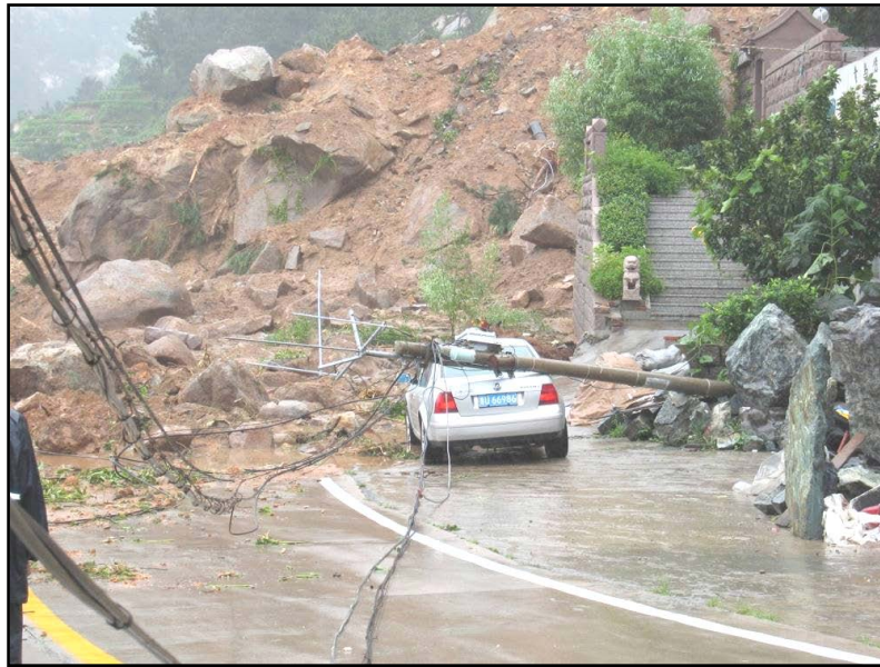
Figure 1. The scene of geological hazards 图 1. 地质灾害现场
