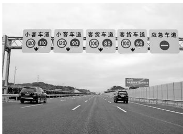
Figure 6. The lane division by the model size (reference case) 图 6. 按车型大小划分车道(参考案例)
