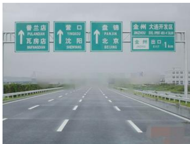
Figure 7. The lane division by the export order (reference case) 图 7. 按出口顺序划分车道(参考案例)
