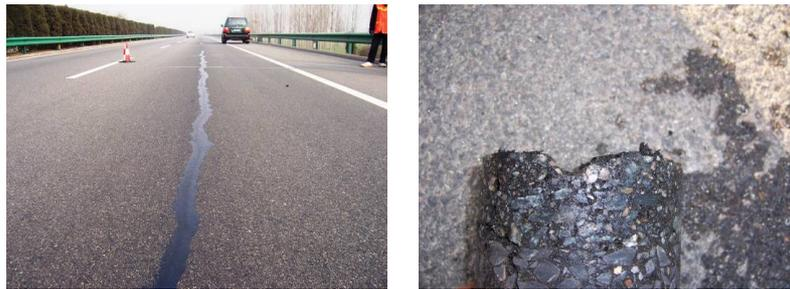
**Figure 5. The longitudinal crack of road surface and core**
