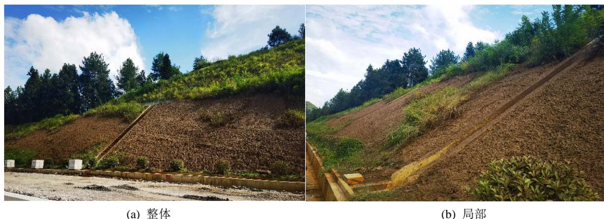
**Figure 5.** On-site photo of the slope after cement-soil sealing treatment
