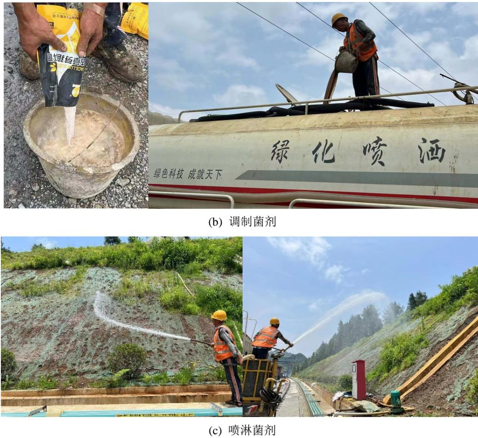
**Figure 3.** Photo of the on-site construction of ecological restoration of coal gangue slope
