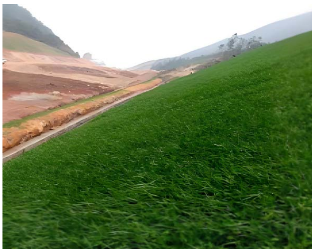
Figure 5. Ecological vegetation blanket 图 5. 生态植被毯
