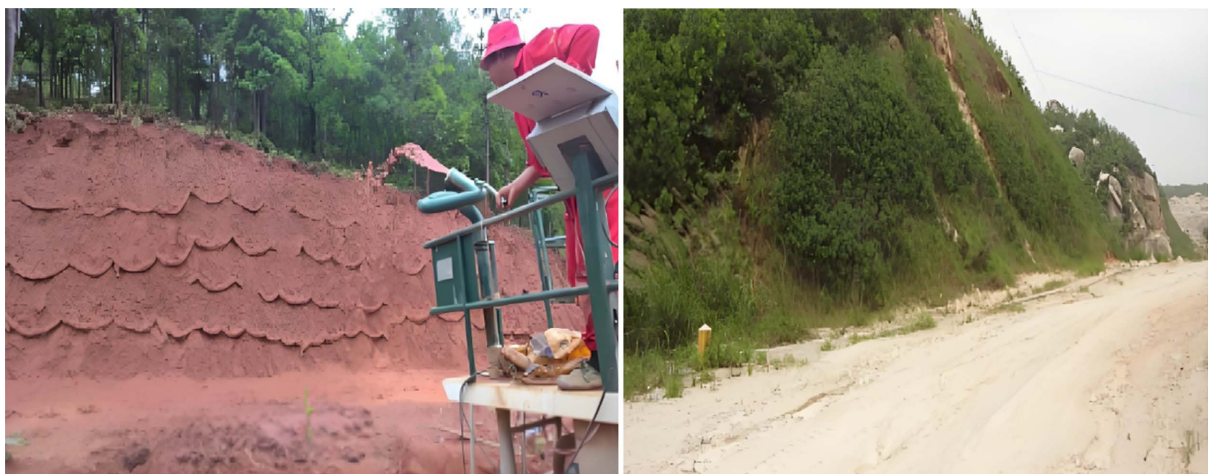
Figure 9. Shotcreting with wire mesh for slope protection 图 9. 挂网喷播护坡
