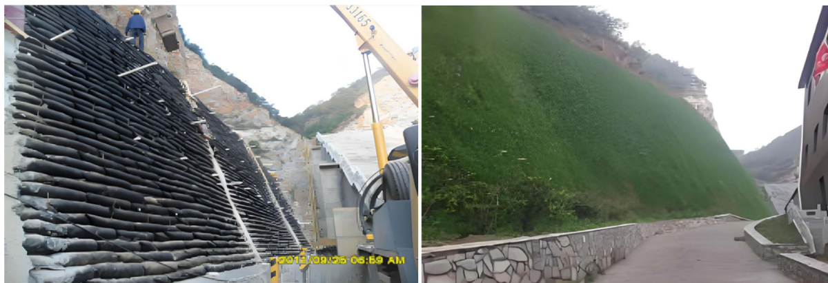
Figure 3. Ecological bag slope protection
