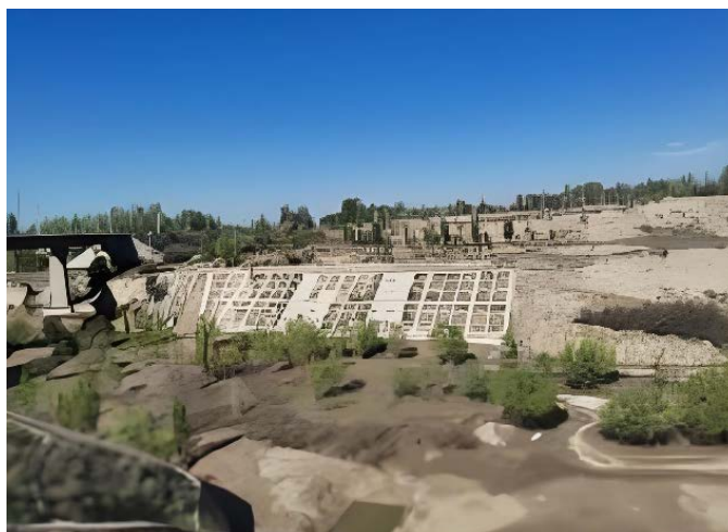
Figure 7. Concrete lattice structure + grass planting measures 图7. 混凝土格构 + 植草措施
