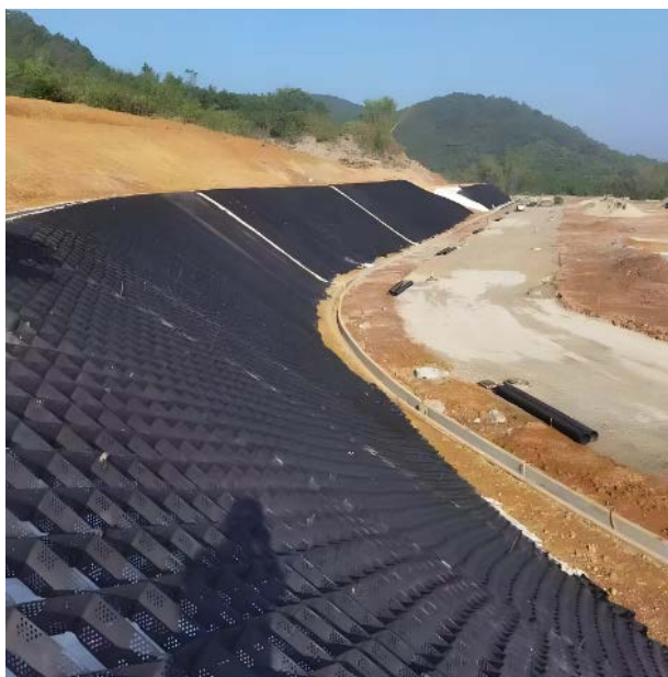
Figure 6. Slope protection with vegetation belt 图 6. 植生带护坡
