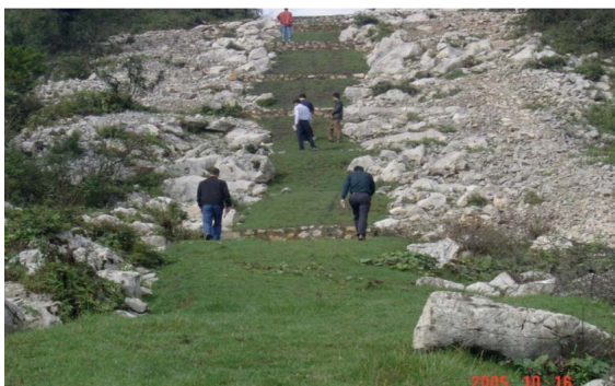
Figure 2. Grass planting slope protection 图2. 植草护坡
