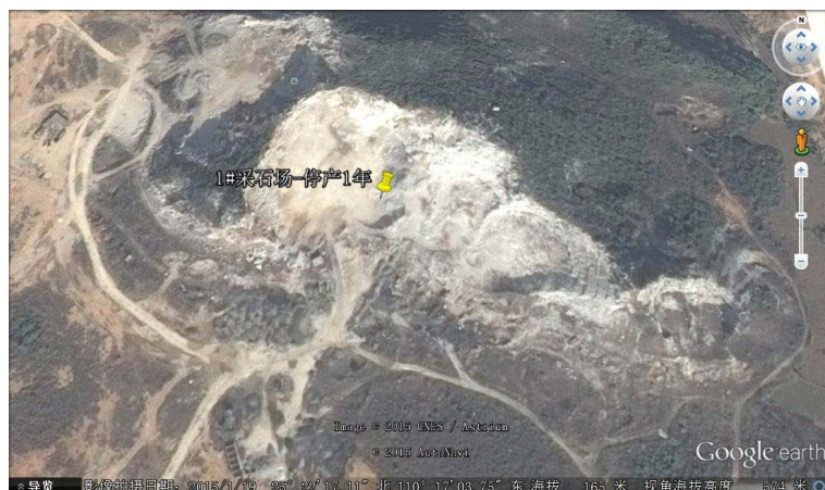
Figure 1. 1# remote sensing image of quarry
