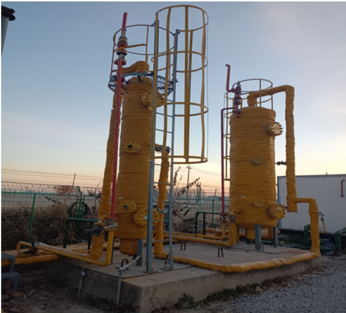
Figure 2. Application of vertical gas-liquid separator 图 2. 立式气液分离器应用
