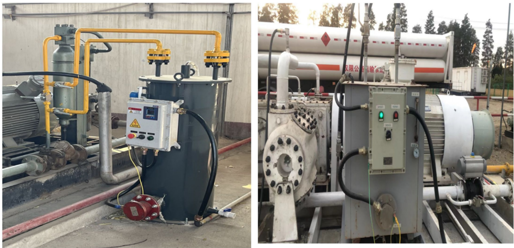
Figure 7. Application of the water-bath rewarmer 图 7. 水浴式复温器应用
