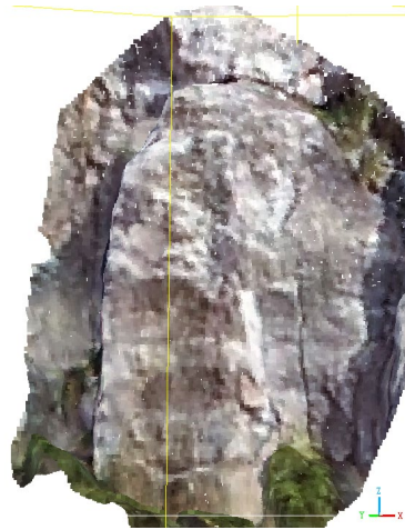
Figure 14. Real-scene point cloud of Unstable Rock 2 图 14. 危岩 2 实景点云
