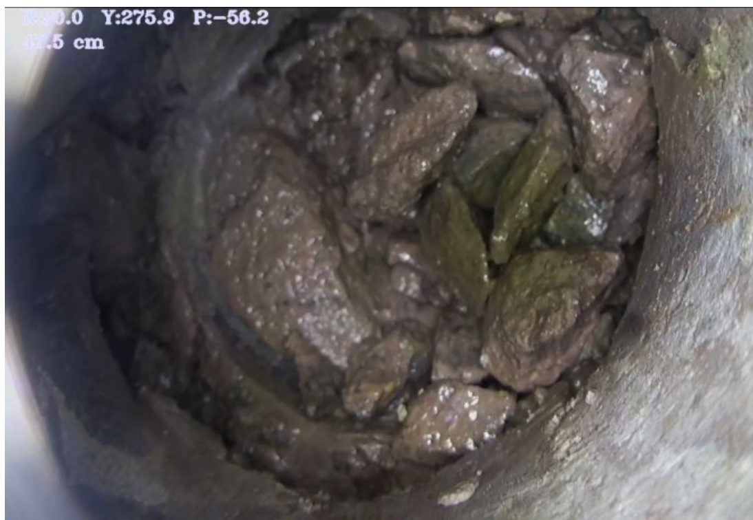
Figure 9. Screenshot from borehole video of ZK1 (within the air-gap anomaly zone)
