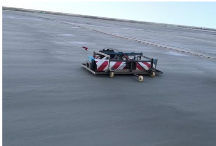
Figure 3. Photo of 3D ground penetrating radar inspection of dams 图 3. 三维探地雷达大坝检测照片
