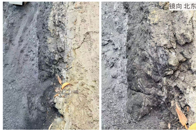
Figure 3. Partial view of fault gouge 图 3. 断层泥局部图
