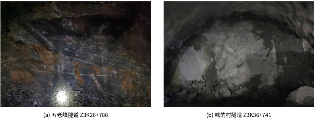
Figure 3. Comparison of tunnel-face geology in the two cases 图 3. 两案例掌子面地质特征对比
