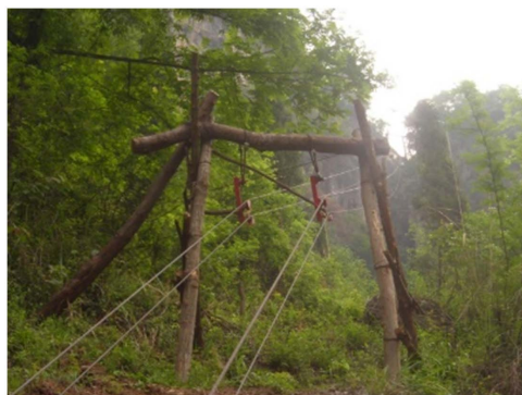
Figure 1. Wooden cableway support 图 1. 木质索道支架
