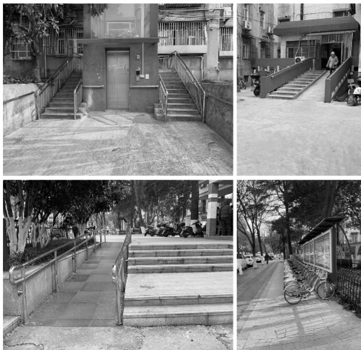
Figure 2. Practice 1 on the renovation of Suojincun Subdistrict 图 2. 锁金村街道改造实践 1
