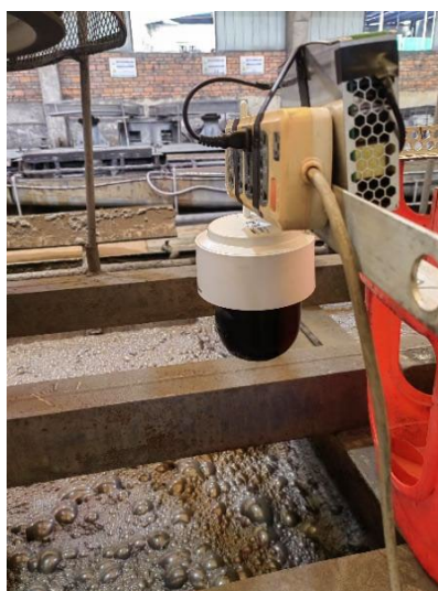
Figure 1. Field installation of the flotation froth image acquisition device 图 1. 浮选泡沫图像采集装置现场安装图
