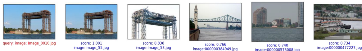
Figure 11. Steel framework interference
