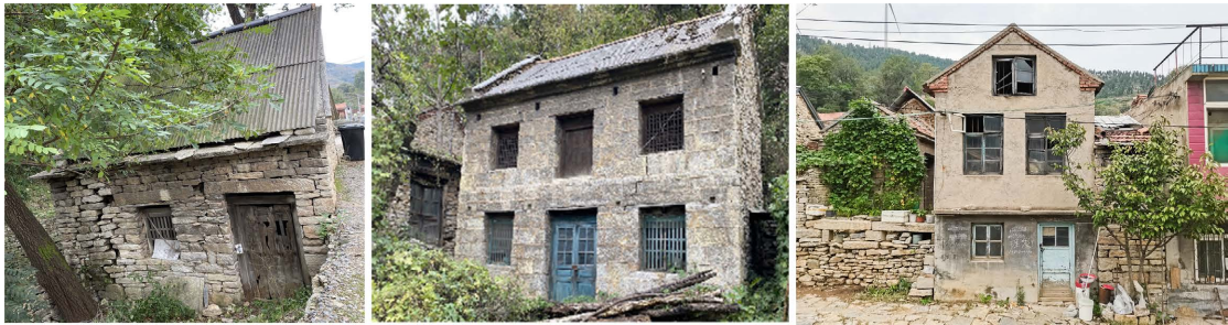
Figure 5. Waste building status 图 5. 废弃房屋现状 ®
