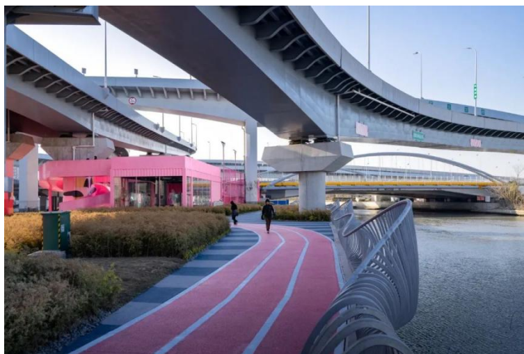
Figure 4. Space under the Zhonghuan Bridge on Beizhai Road, Shanghai 图 4. 上海北翟路中环桥下空间 ④
