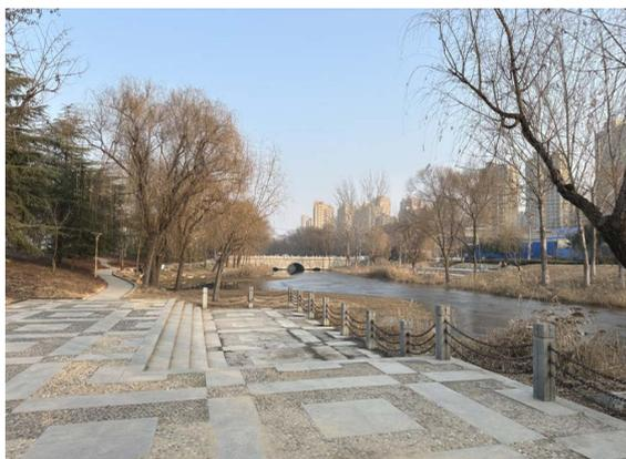
Figure 4. The hydrophilic platform position is too low
