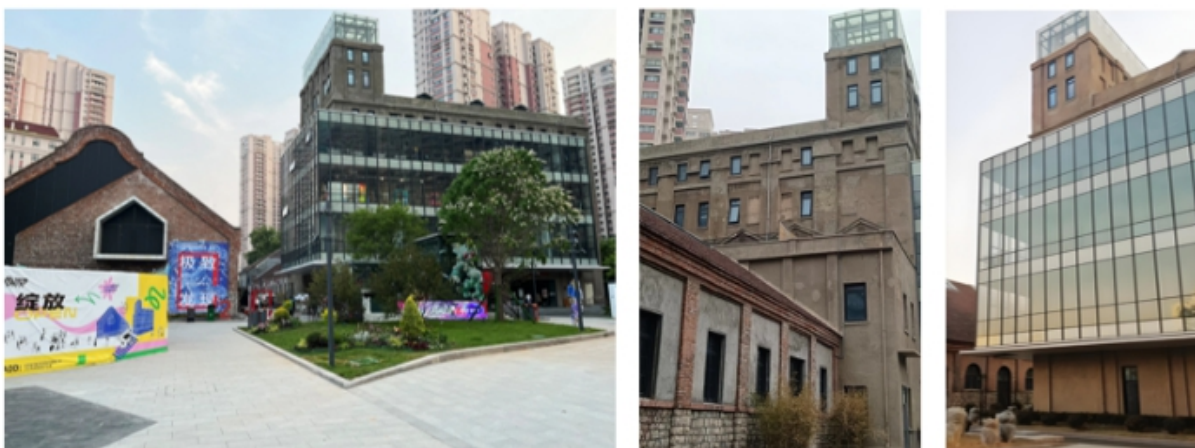
Figure 2. Current situation of the powder mill building
