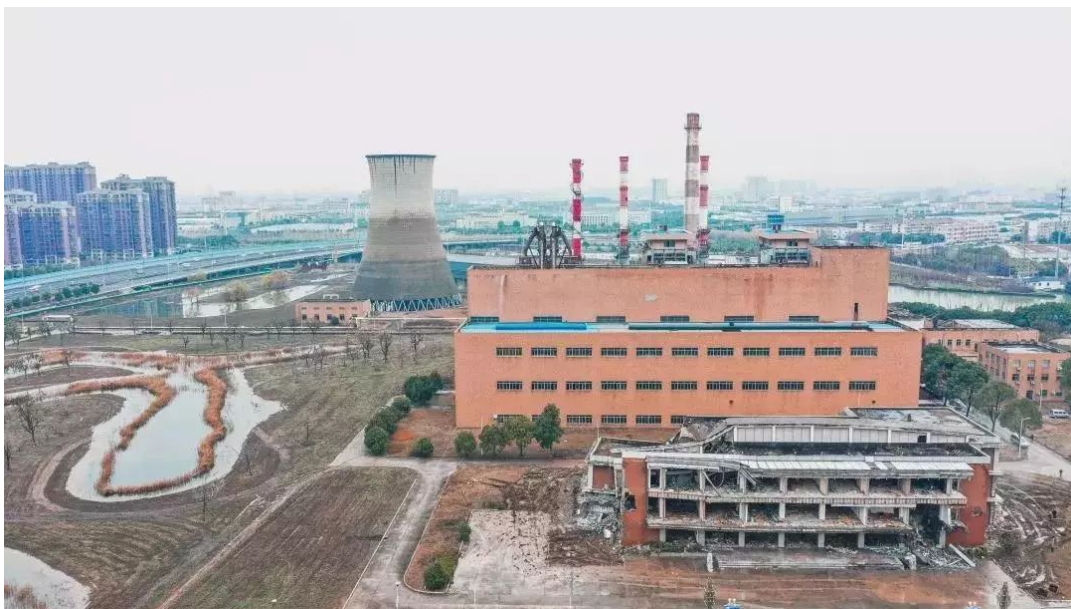
Figure 1. Aerial view of the power plant 图 1. 电厂现状航拍 ①
