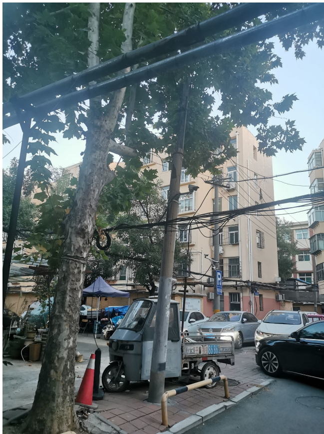
Figure 3. All facilities are seriously aging 图 3. 各设施老化严重 ①
