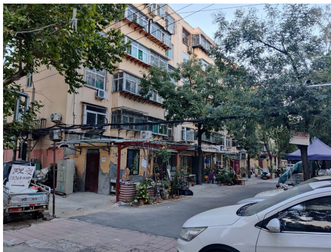
Figure 1. There are potential building safety risk 图 1. 存在建筑安全隐患 ①
