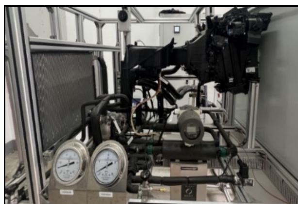
Figure 2. CO 2 heat pump air conditioning system testing
