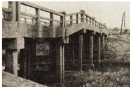
Figure 1. Bridge frost heave damage
