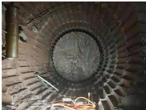
Figure 6. Water drilling and static blasting hole formation diagram
