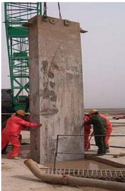
**Figure 5.** Schematic diagram of the installation of the guide plug-in plate
