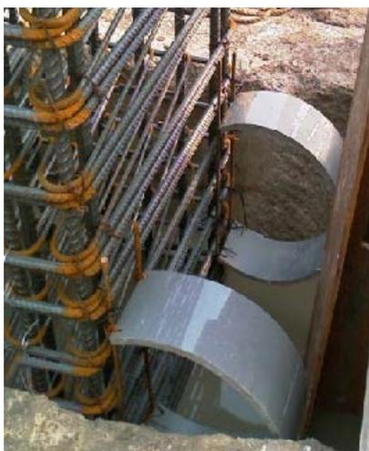
**Figure 4.** Schematic diagram of installation location of PVC pipe
