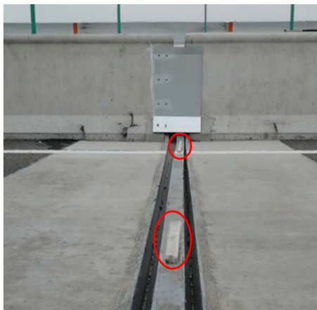
Figure 10. Simulation of height difference of expansion joint
