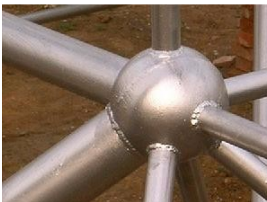
Figure 4. Hollow sphere joint 图 4. 空心球节点
