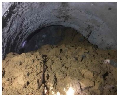
Figure 1. Tunnel mud inrush and collapse
