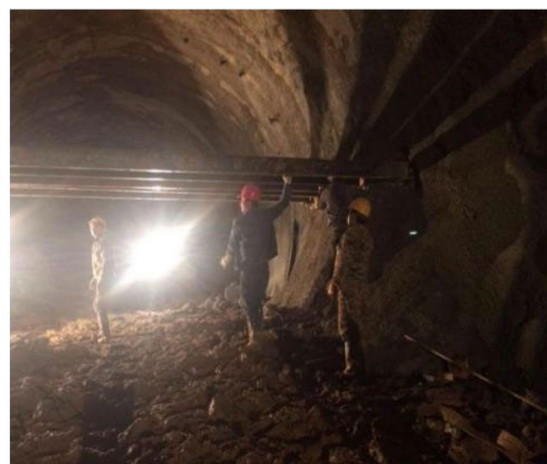
Figure 12. Reinforcement of collapsed area with transverse supports
