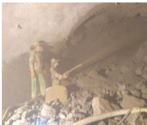
Figure 11. Shotcrete and anchor bolt sealing of collapsed soil mass
