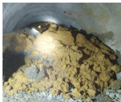
Figure 2. Tunnel karst cave mud inrush and collapse
