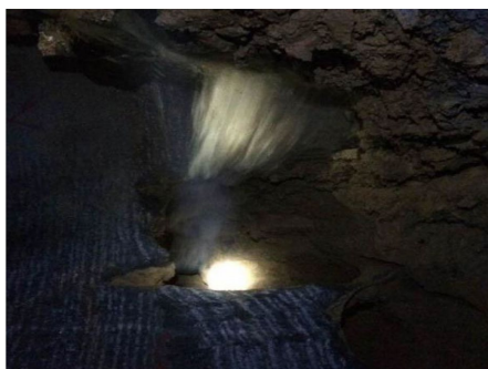
Figure 3. Tunnel karst cave water inrush and collapse
