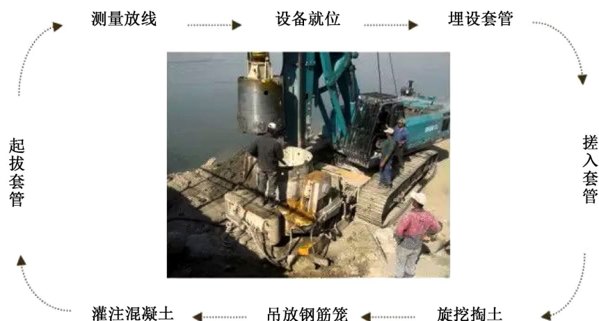
Figure 7. Process flow chart of the pipe ramming method construction 图 7. 搓管法施工工艺流程图
