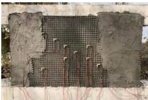
Figure 4. Masonry wall paved with polypropylene mesh composite polymer mortar 图 4. 聚丙烯网复合聚合物砂浆铺设的砌体墙
