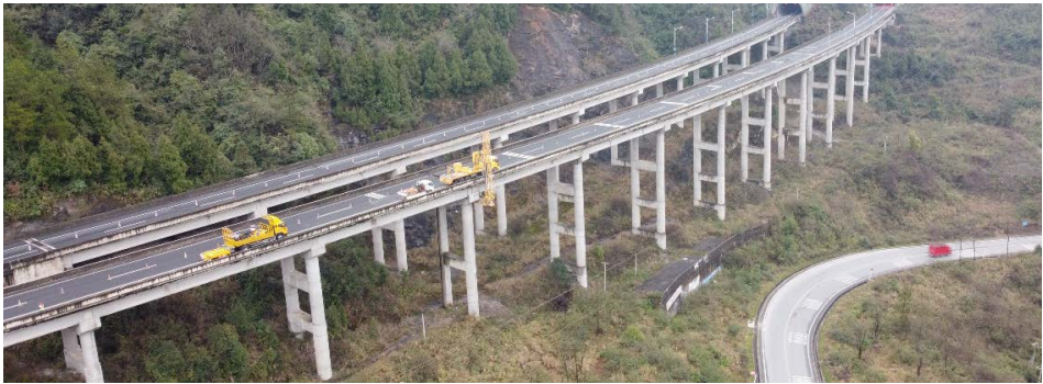
Figure 15. A highway bridge in a mountainous area of Guizhou Province 图 15. 贵州某山区高速公路桥梁
