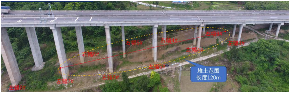
Figure 9. Diagram of the filling soil range under the bridge 图 9. 桥下填土范围图示
