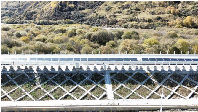
Figure 1. Panoramic view of Jiuma Expressway cadmium telluride power generation intelligent snow and ice melting system 图 1. 久马高速碲化镉发电智能融雪化冰系统全景图
