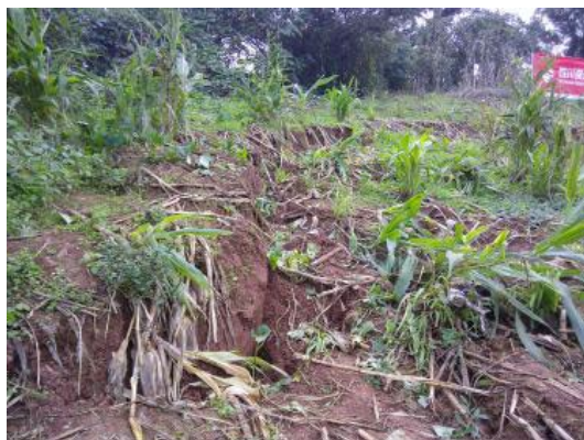
Figure 6. right boundary (shear crack) 图 6. 右侧边界(剪切裂缝)
