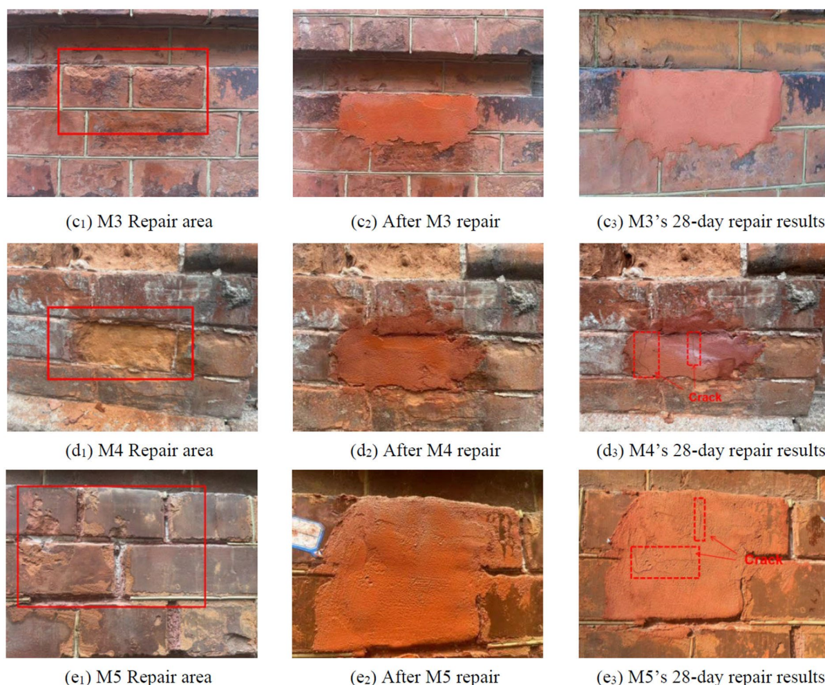
Figure 11. Comparison before and after repair and at 28 days wall condition
