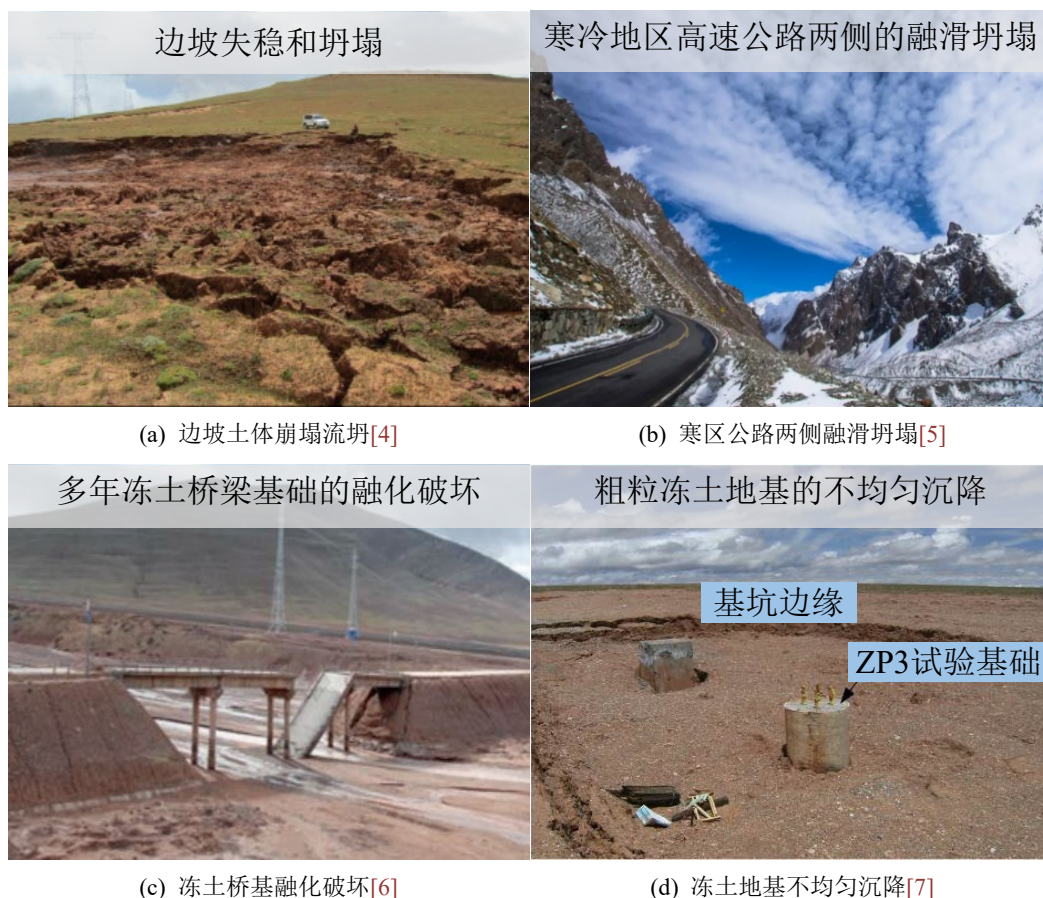
Figure 1. Engineering disasters in frozen soil area
