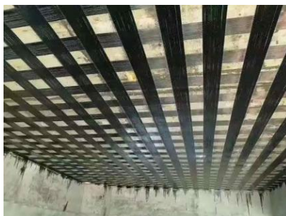
Figure 4. Schematic diagram of the structure of the BFRP reinforced floor slab
