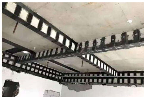
Figure 3. Schematic diagram of the structure of the BFRP reinforced beam
