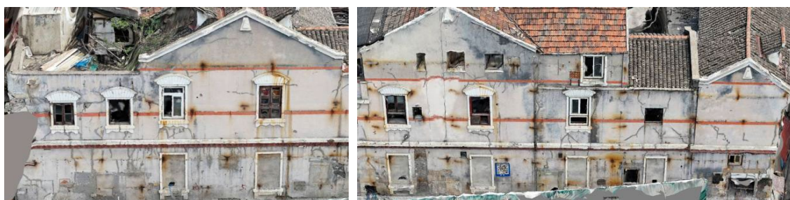
Figure 8. Tilt photography model of exterior facade
